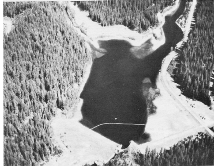
Source: Oregon National Guard, 1981-82. View looking north.
